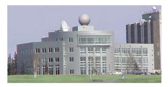
**Figure 1.** UAF-GINA's X-band receiving station antenna is inside the radome in the center of the photograph. The large, fixed dish to its left is the NWS Fairbanks WFO's NOAAport antennna. The small radome in the upper right holds an L-band antenna.
